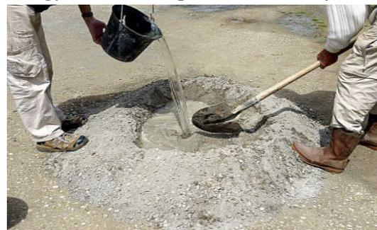
**Figure: Adding water to cement mix**
