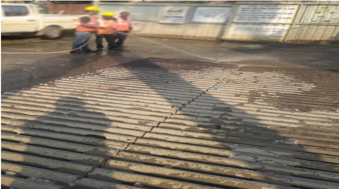
**Figure .8 Daily Washing of Truck Wheel Wash Tracker to Remove Muck Generated During Construction Work.**
