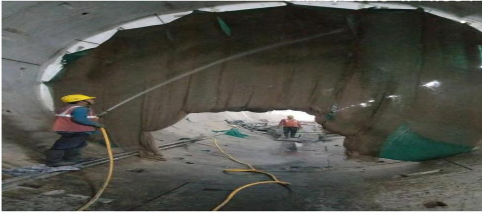
**Figure 4. Water Curtain Used during Construction to Minimize Air Pollution**
